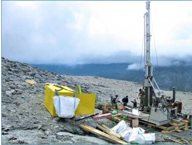
Drilling on exposed eudialyte layers
